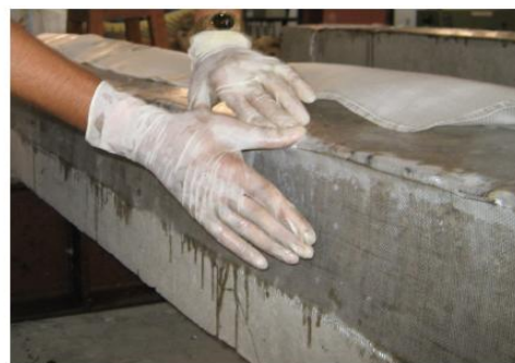
FIG 5 FIXING OF GFRP SHEET ON THE BEAM
