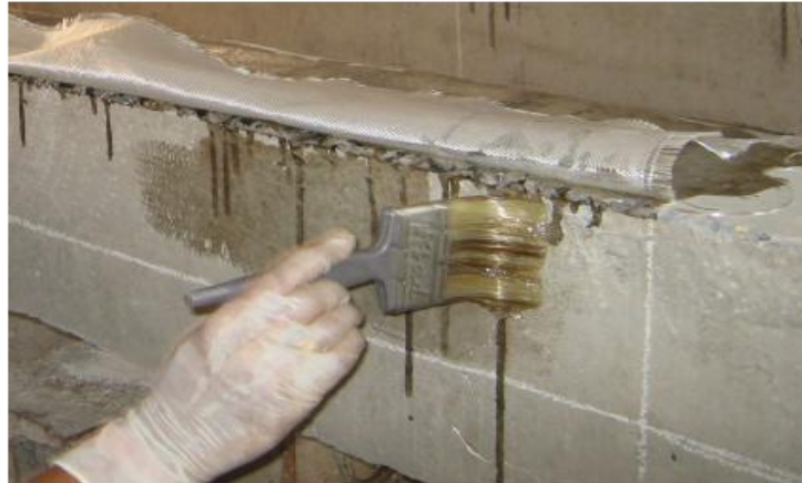
FIG 5 APPLICATION OF EPOXY AND HARDENER ON THE BEAM
