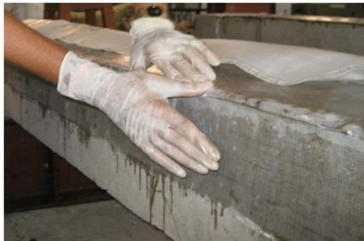
FIG 6 FIXING OF GFRP SHEET ON THE BEAM
