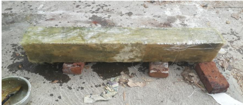
FIG 14 GFRP U-WRAPPING ON THE BEAM
