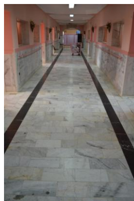
FIG. 14: THE MAIN CORRIDOR OF UNIT NARVAN2, NEGARANDE
